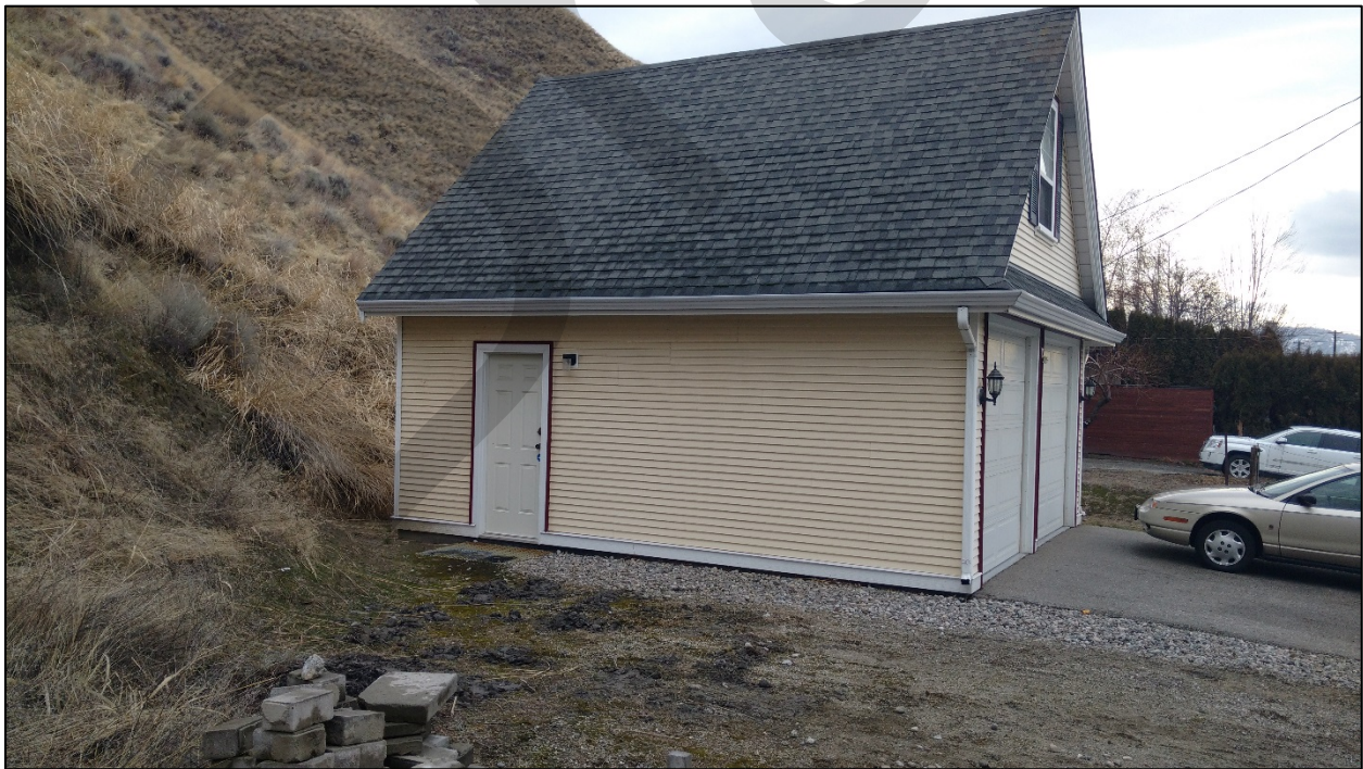
Figure 5: North View of Existing Garage
