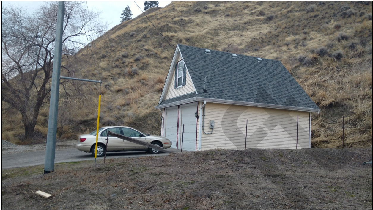
Figure 6: South View of Existing Garage
